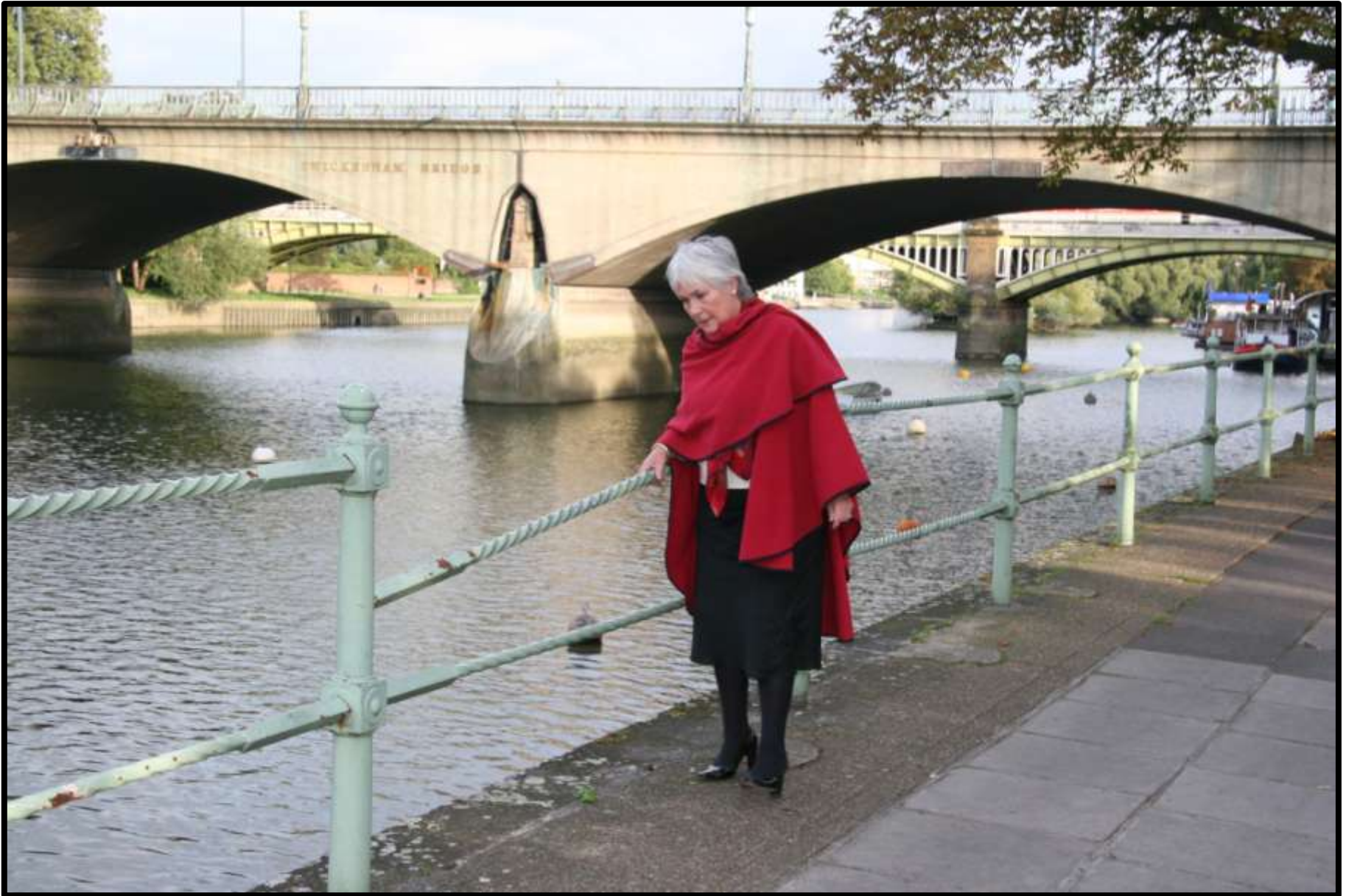
Inspecting the old broken Edwardian cast iron railings along St Margaret's Riverfront 29 Sept 05 before works started with X Cllr Annie Hambidge
