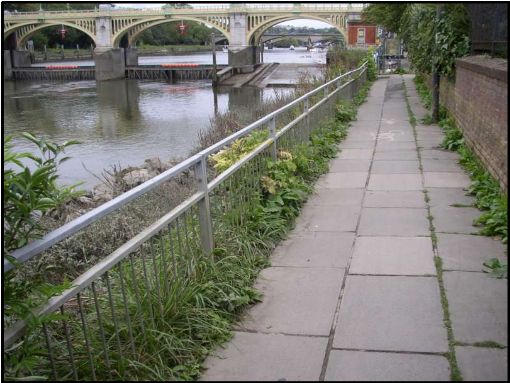
In many places the Edwardian cast iron railings along St Margaret's Riverfront had been replaced with modern galvanised railings in the 1980's as seen here on 17 Sept 2004 as one looks towards the grade II* Richmond Lock.
