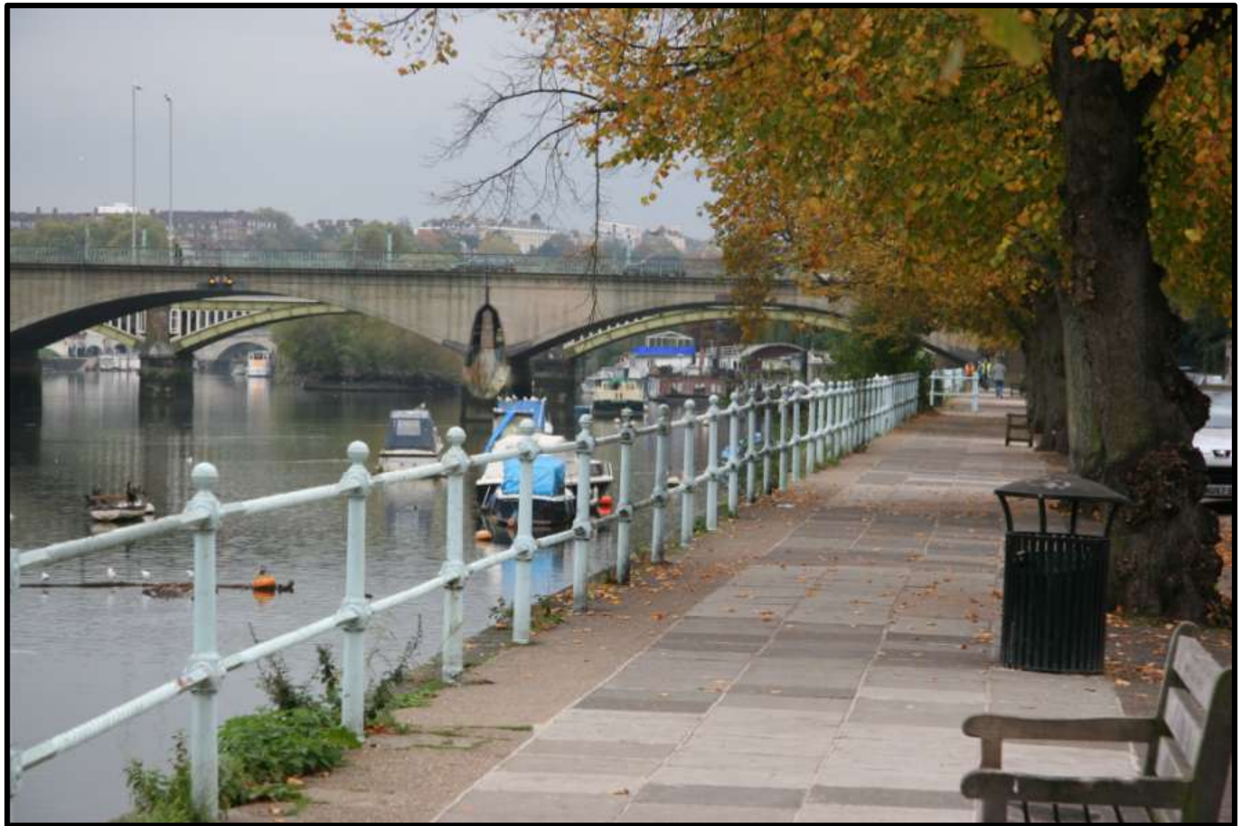
The restored Edwardian cast iron railings along St Margaret's Riverfront and Isleworth Promenade after works completed with new street furniture and interpretation. Nearly a mile of cast iron railings were restored as part of the works.
