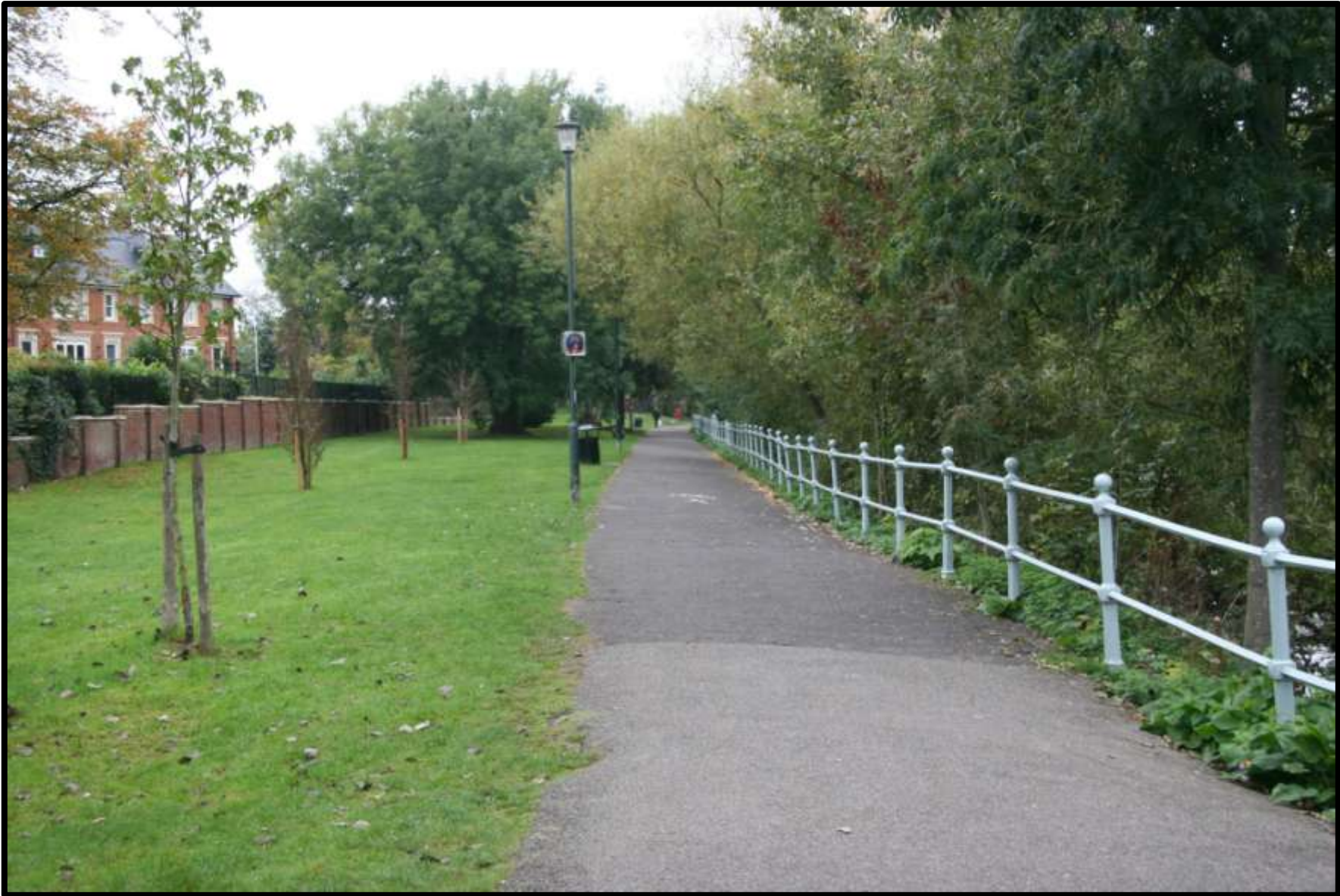
The restored Edwardian cast iron railings along Isleworth Promenade after works completed with new street furniture in background and new landscaped areas with trees planted. Nearly a mile of cast iron railings were restored as part of the works.
