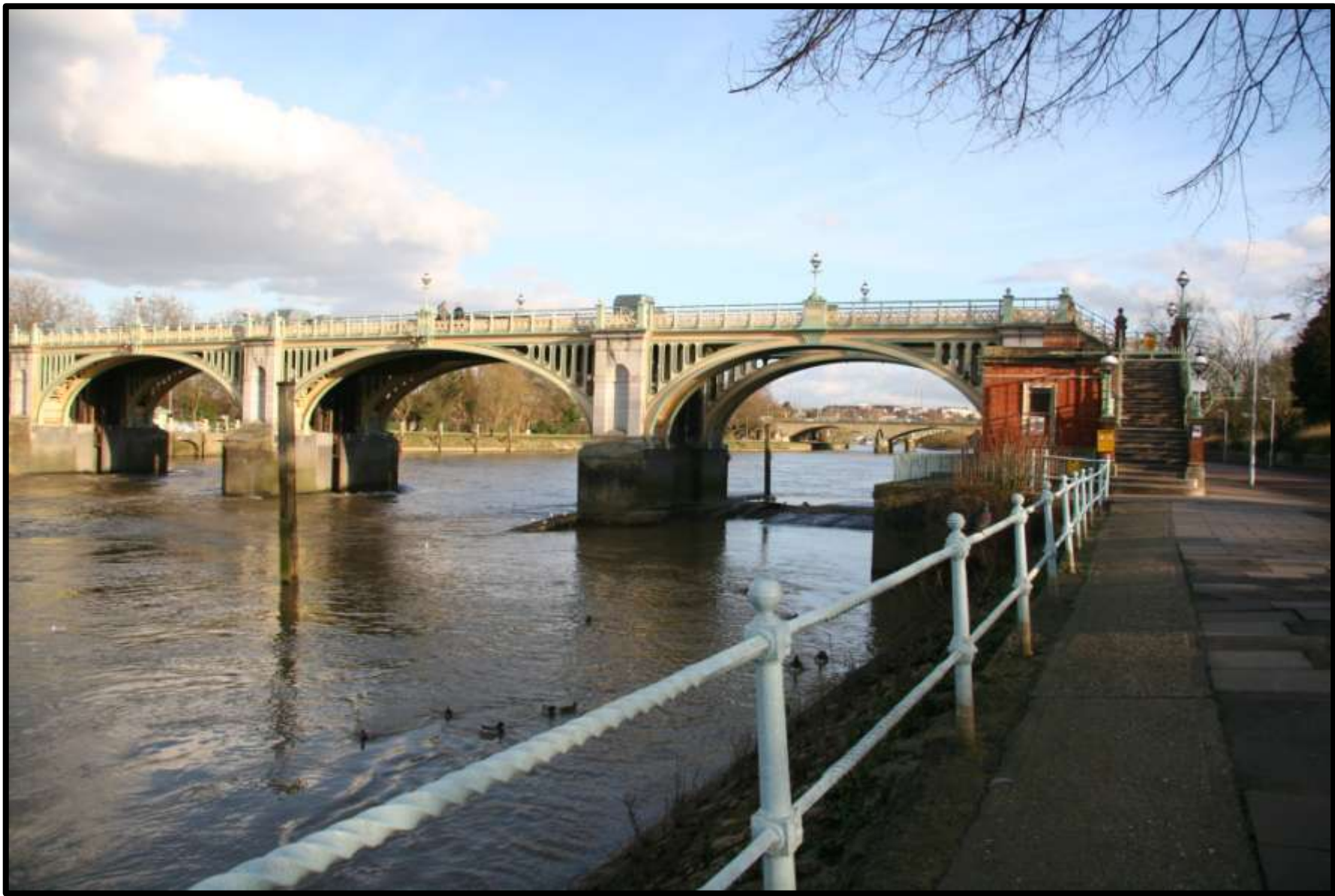
The restored Edwardian cast iron railings along St Margaret's Riverfront and Isleworth Promenade 26 February 2007 looking to the grade II* Richmond Lock.
