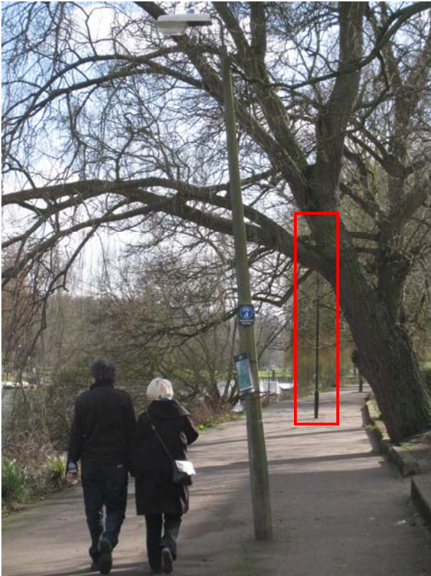
Figure 2 Showing current street lights on the Warren Footpath. Note non uniformity of lights and placement in the middle of the footpath.
