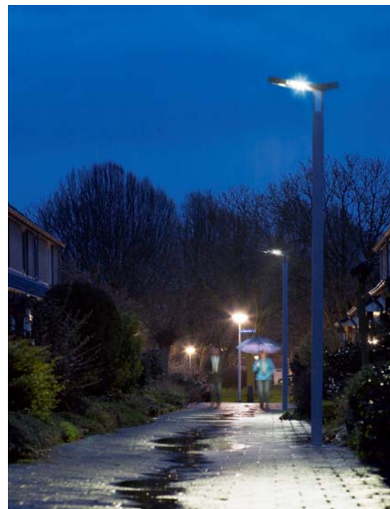
Figure 5 showing proposed lighting as used at a site in Europe.
