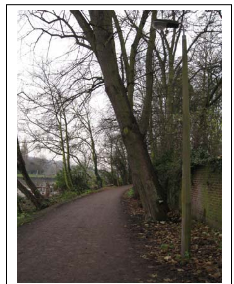
Figure 6 Street light with concrete column
