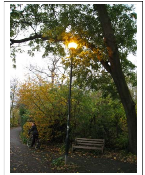
Figure 5 Metal column with spherical fixture. Light is on during daylight hours when not needed
