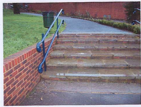
Sample steps with York stone treads and brick risers and handrails for Rotary Gardens as in Riverdale Gardens
